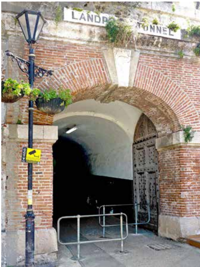
The Landport Tunnel, giving access to the Landport Gate
